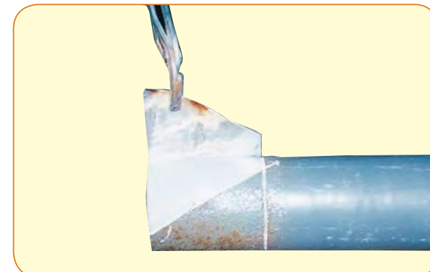
3 Peel off the FRP layer by pinching it with pliers or the like.
