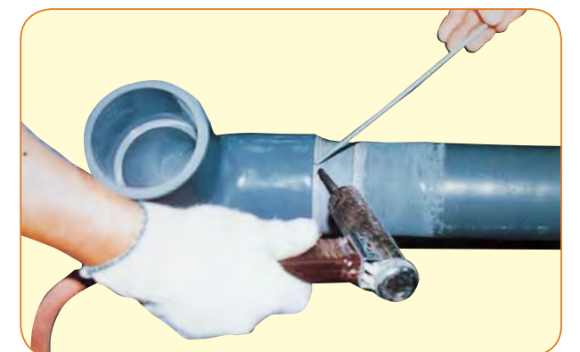
6 Wipe off any adhesive sticking out, and weld the parts.
